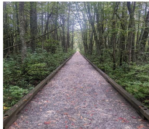
Estell Manor Park Boardwalk
